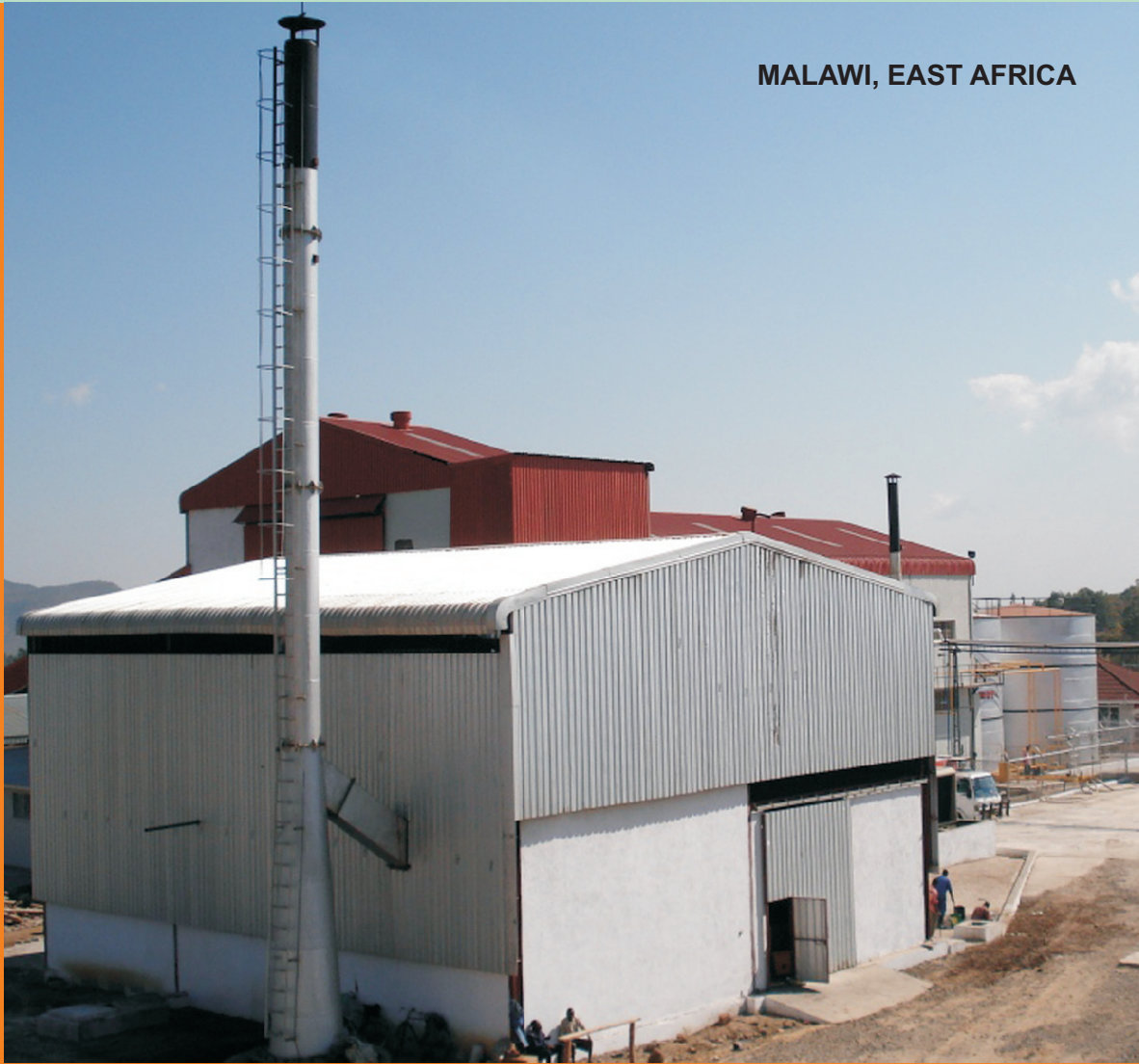
SPECTEC'S 120 tpd continuous refinery ( out side )
